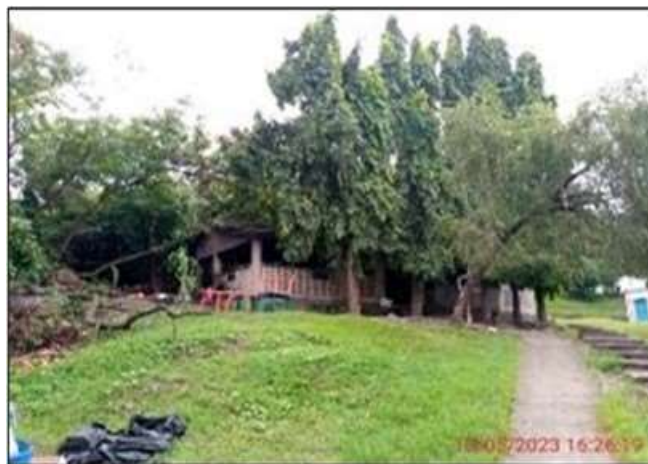
Plate No. 2.3-1: Kitchen Building, Paved Walkway short grass in the surroundings
