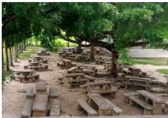
Plate No. 2.3-4: Circular and Rectangular Concrete Desks inside he proposed workshop and laboratory construction site.
