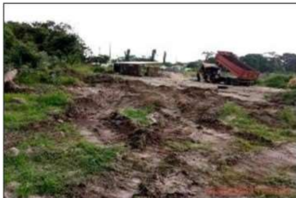
Plate No. 2.3-3: Workshop Building under construction on the north-western boundary.
